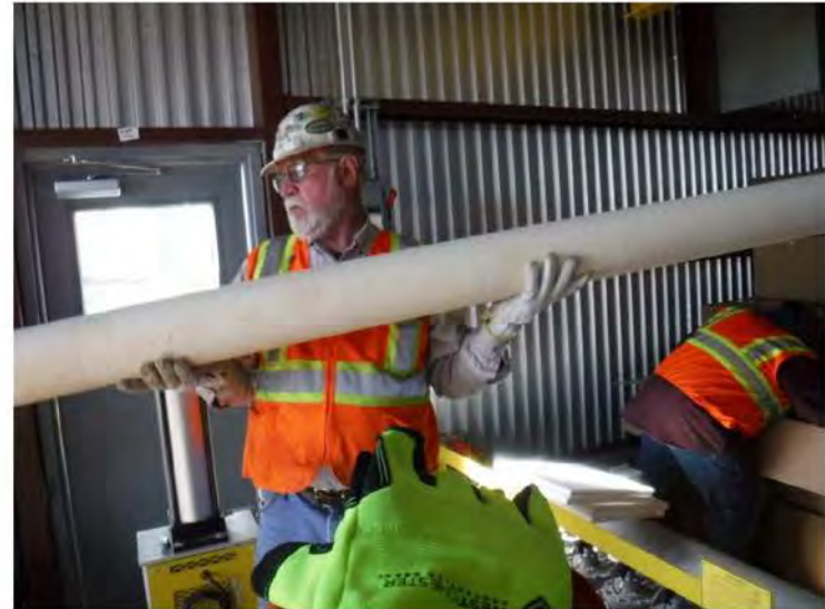
Moving ceramic filters into filter housing
