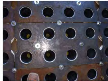
Close-up of seal plate covers
