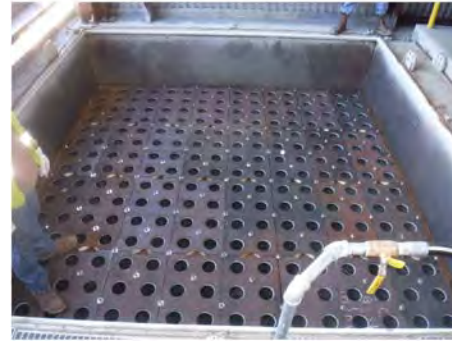
Compartment filled with ceramic filters
