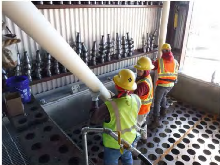
Positioning ceramic filter for loading
