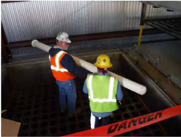
View of full 3-meter ceramic filter length
