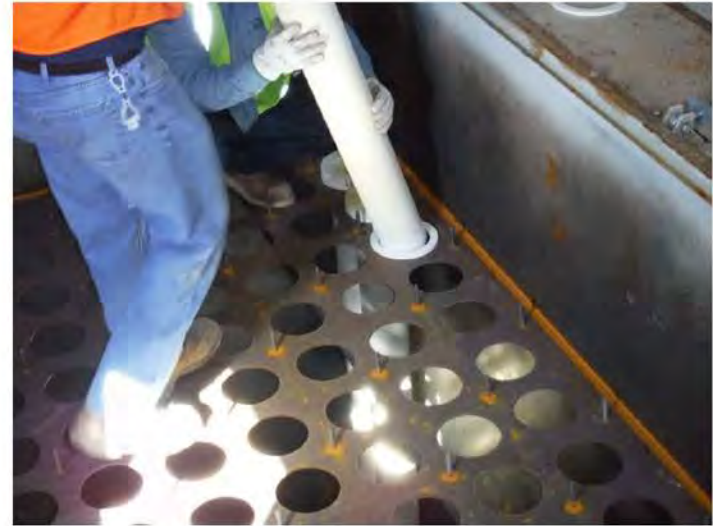
Ceramic filter carefully placed into cell plate
