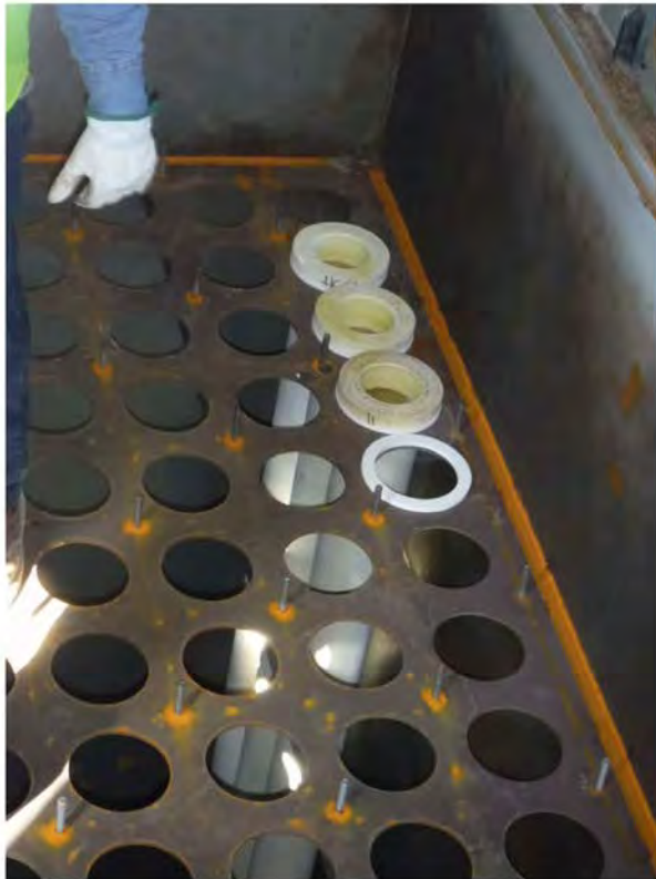
Ceramic filters loaded into cell plate
