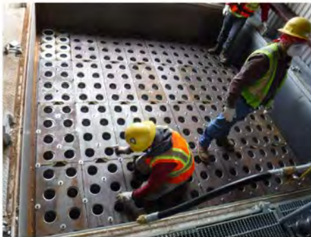
Inspection of seal plates
