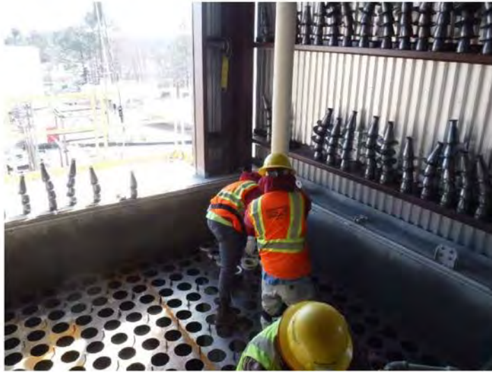
Ceramic filter turned vertical for loading
